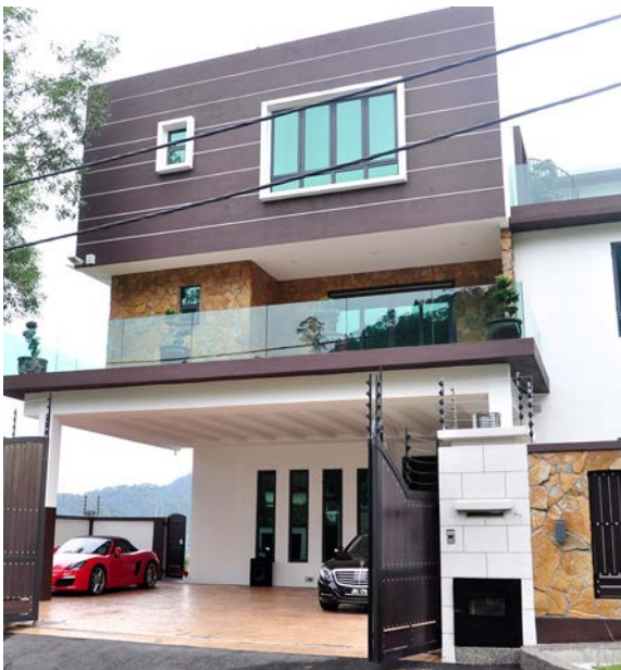
TEMPLER VILLA KUALA LAMPUR - (MALAYSIA)
